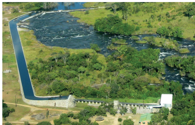
The 750 kW Zengamina run-of-river mini-hydro scheme, in North West Province, Zambia, is a privately developed community initiative that serves a hospital, several schools, small businesses and households, about 550 customers in total, who are more than 100 km away from the national grid.
