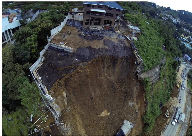
Landslides caused by torrential rains are increasingly common in Central America. Above, a landslide in 2013 onto a highway in Guatemala City.
