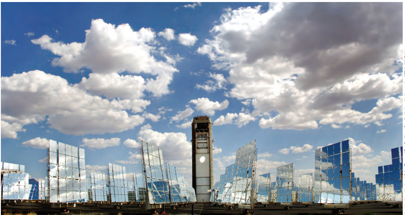
New Mexico – National Solar Thermal Test Facility at Sandia National Laboratories @Flickr/NNUSAnews
