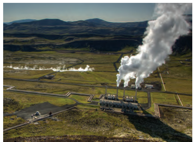
Iceland – geothermal power plant ©Flickr/Scott Ableman
